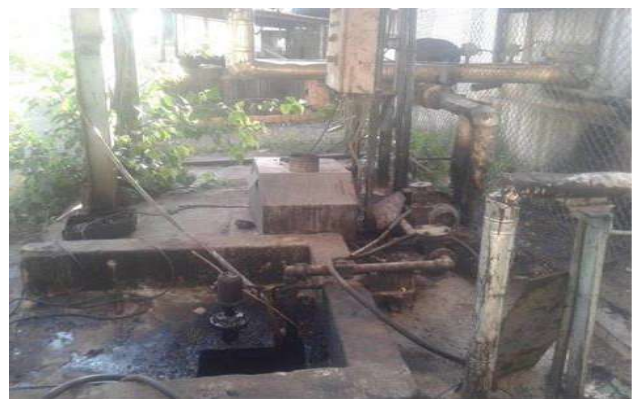
Picture 26 – Waste oil management
